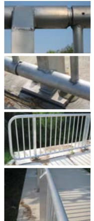
Fabbed 2" SCH 40 Pipe 3.75" between picket walls
